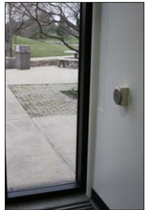
At top right, an automatic door opener for disabled students goes from the ground to the waist-height for a walking user. At bottom right, the button to door opener outside of the Student Union. Buttons going to the ground can be bumped by a wheelchair. Reaching a waist-height button can be impossible for some students in wheelchairs.
