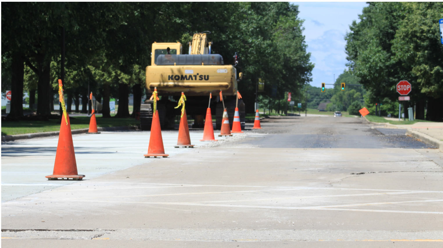
Photos by Regina Ivy/Co-Editor of The Lamp Crews block off a lane of traffic on R.L. Poorman Drive heading out of campus. Construction crews repaved the main roadways on the main campus and paved a gravel parking lot in Taylorville this summer.
