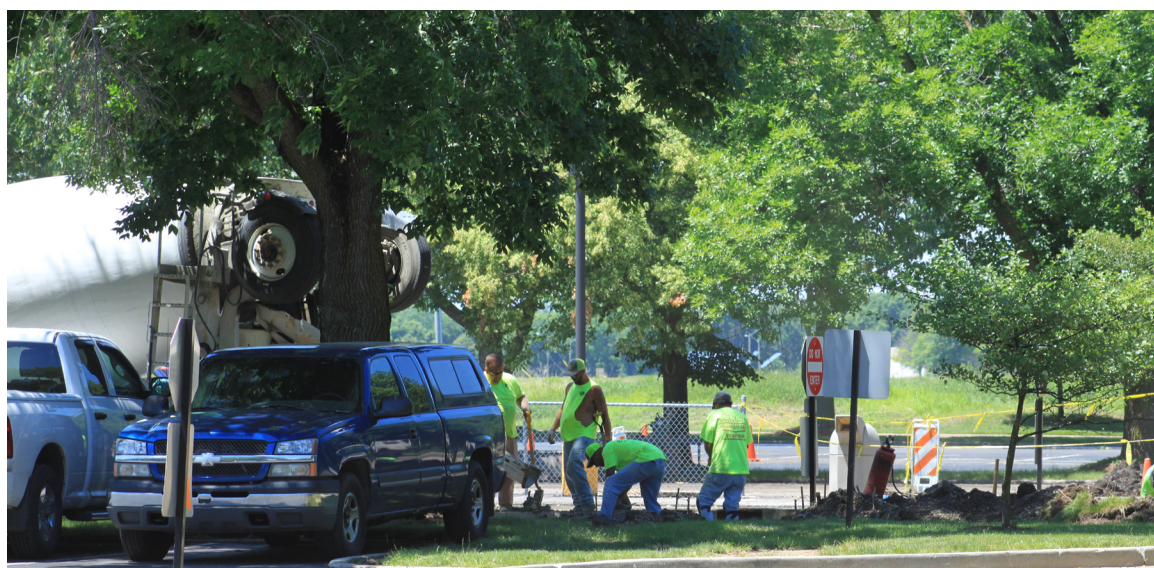
Construction workers replace curbs in the parking lot at the main campus over the summer.
